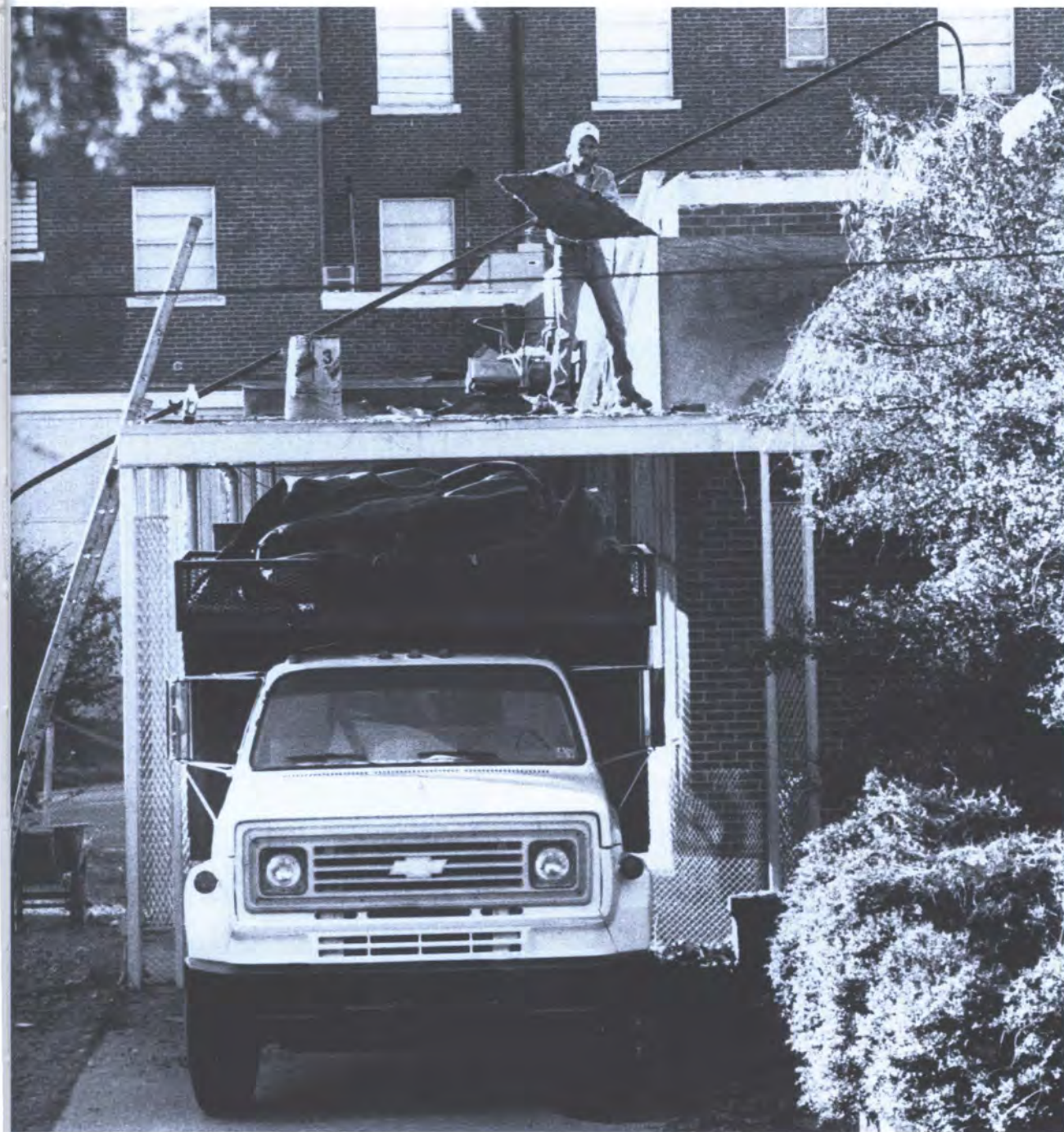
Roofers remove the old shingles on the coffeshop roof. (photo by Kim Bumstead)
